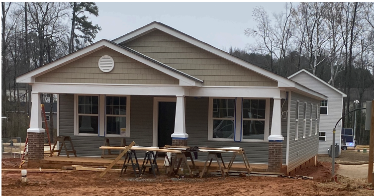
House Number 38 Completed
